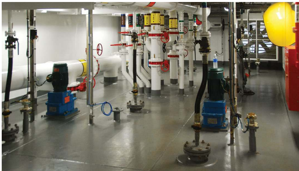
Installed Model 20 agitators on an oil rig
